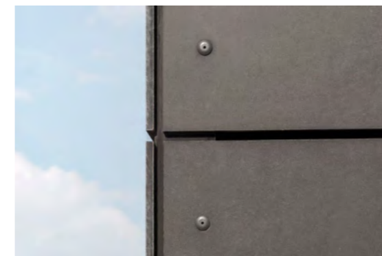
Visible mounting of the fibre cement panels with coloured rivets
