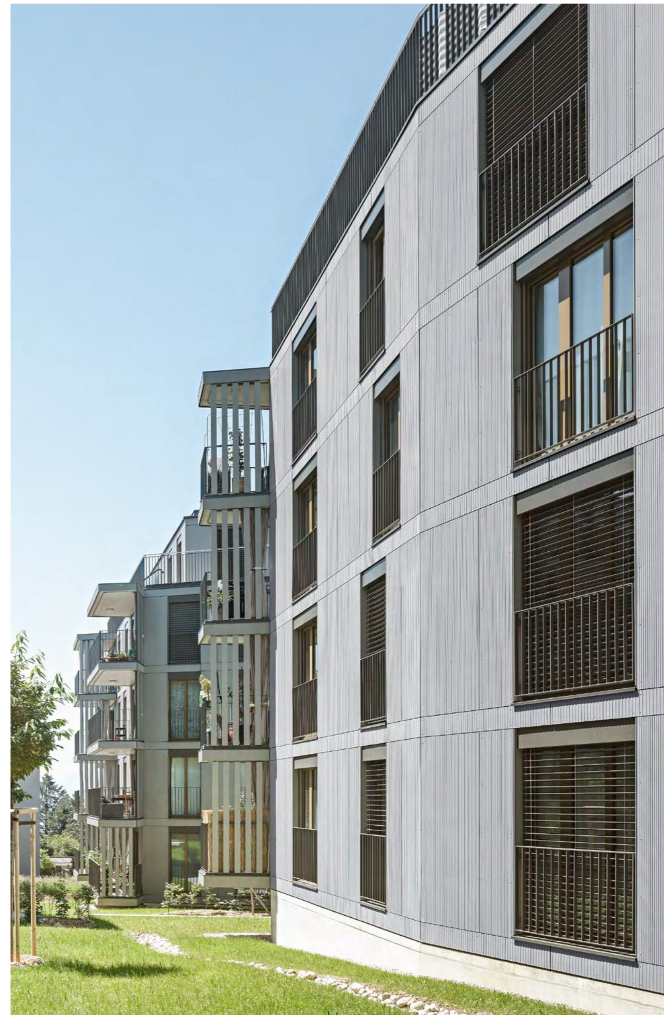
Fiches Nord, Lausanne, Switzerland. Architect: Züst Gübeli Gambetti Architektur und Städtebau AG, Zurich, Switzerland. Photographer: Roger Frei, Zurich, Switzerland.
