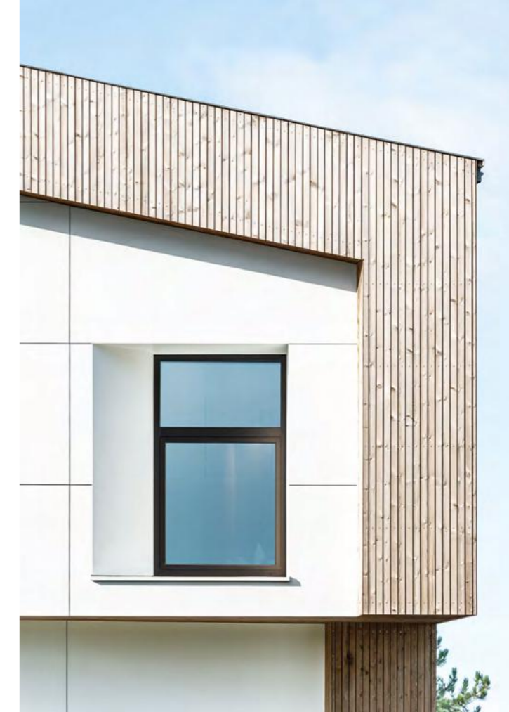
Invisible mounting with the Swisspearl Sigma 8 Pro system
