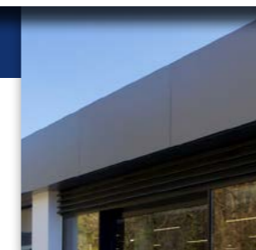
Vitrabond FR Core Vitrabond offers a fire retardant (FR) mineral compound core as standard, offering a fire rating of B-s1,d0.
