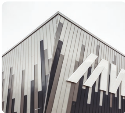
Fibre cement rainscreen panels: Ice Arena, Wales
