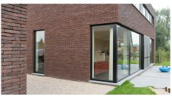
VETAbric+ is a unique click system to create seamless brick panels. By eliminating the traditional grouting process, the overall look is pure and dirt free, with slimmer joints and slimline bricks.
