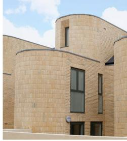
VETAbric by VETA France, have created the thinnest brick slip cladding solution with an adaptable insulated backing panel. Offering a huge range of brick colours and texture options, VETAbric is a lightweight rigid solution, making it easy to install in all weather conditions.
