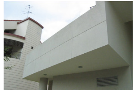
Building services enclosure with exterior paint finish
