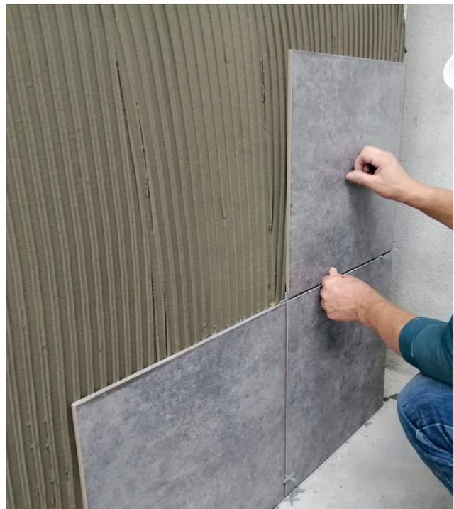
Tile application on SECOLITE® Cement Board
