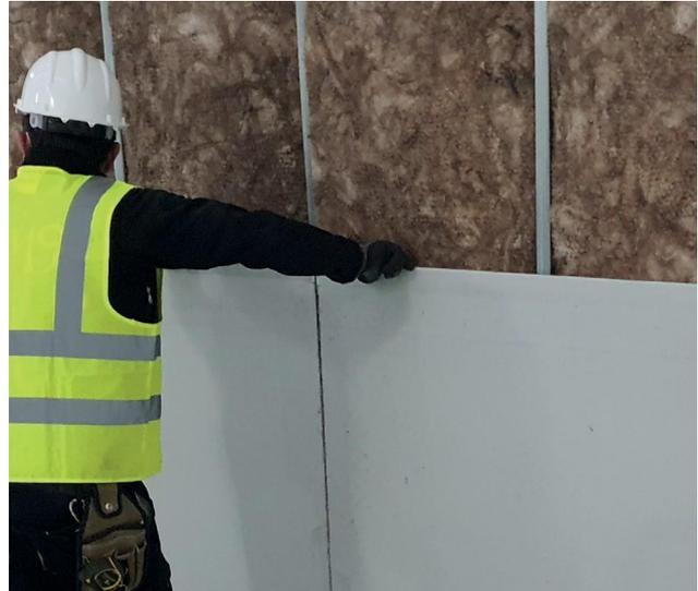
Horizontal installation of SECOLITE® Cement Boards
