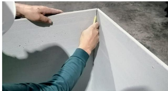
Snap and cut the mesh through on the reverse
