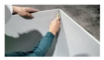
Snap and cut the mesh through on the reverse
