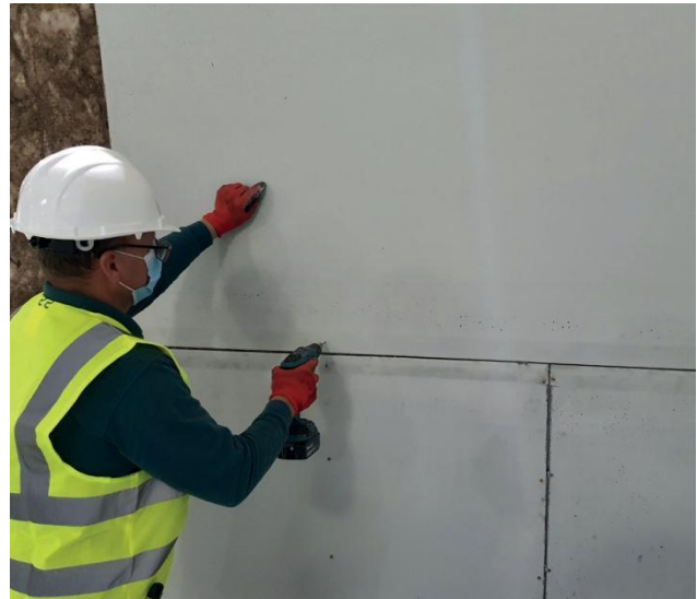
Horizontal installation of SECOLITE® Cement Boards
