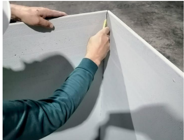
Snap and cut the mesh through on the reverse
