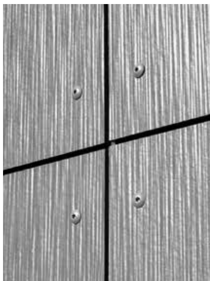
Hardie® Panel Screw Fixing
